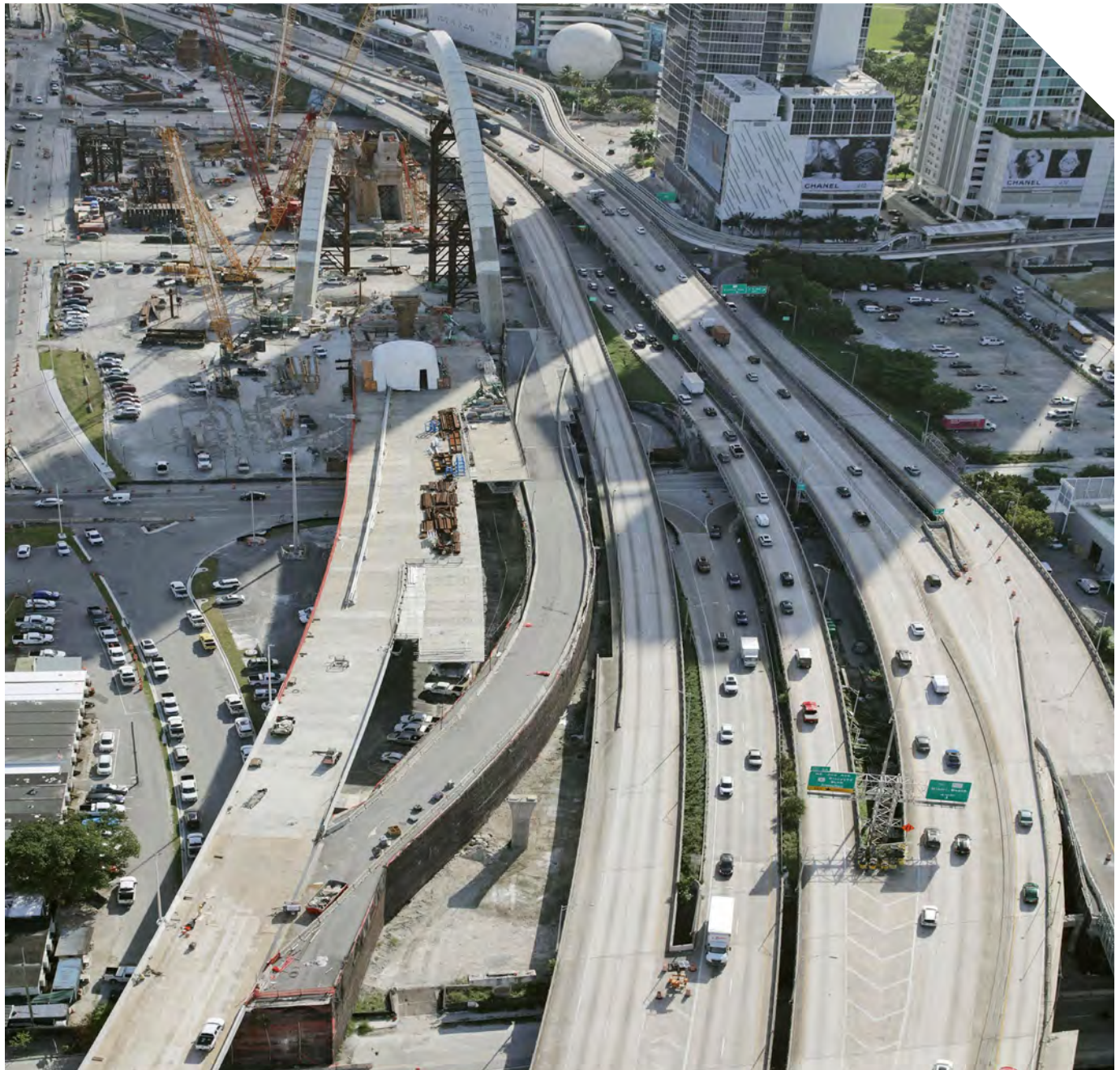
The I-395 Bridge Project.
