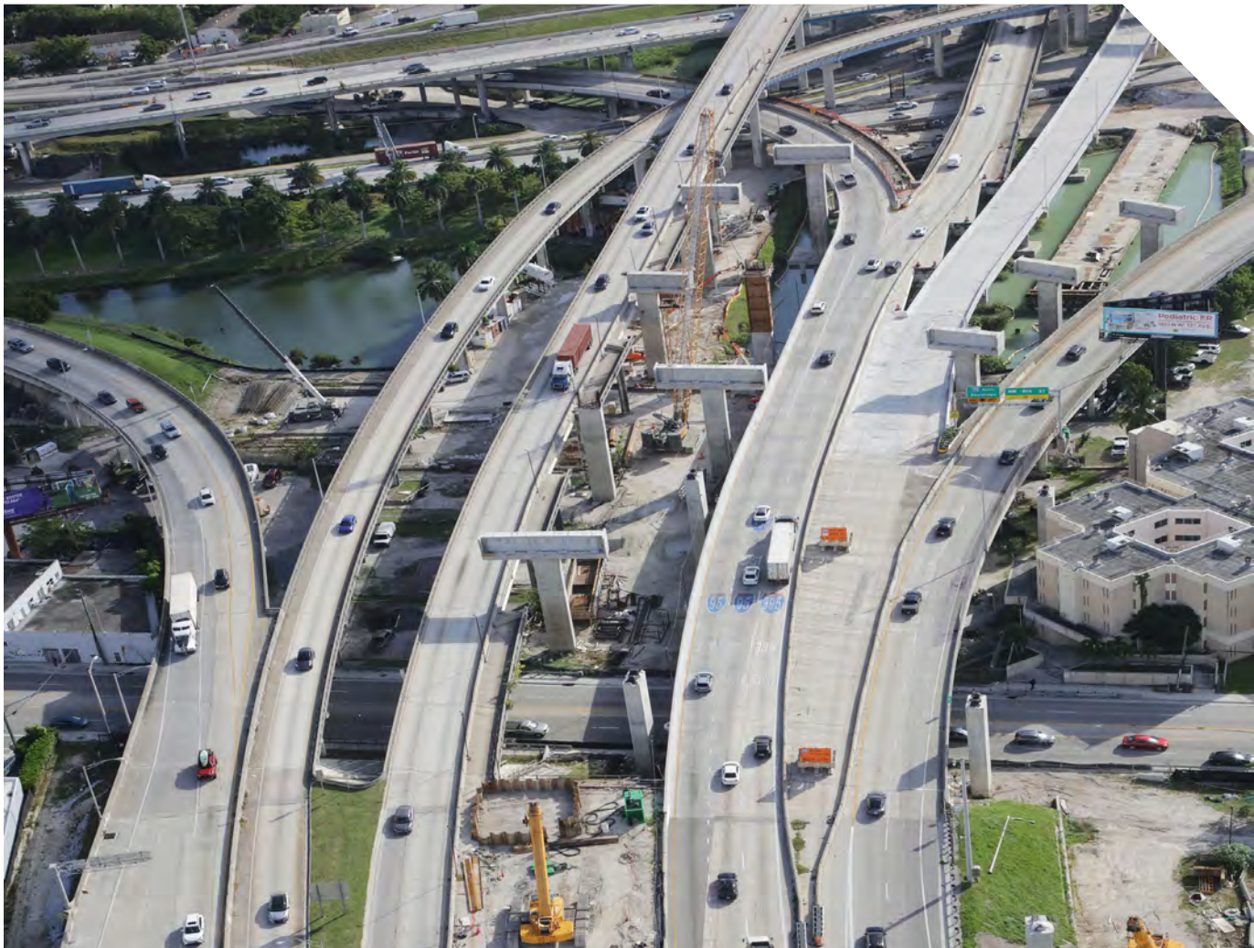
The I-395 Bridge Project.
